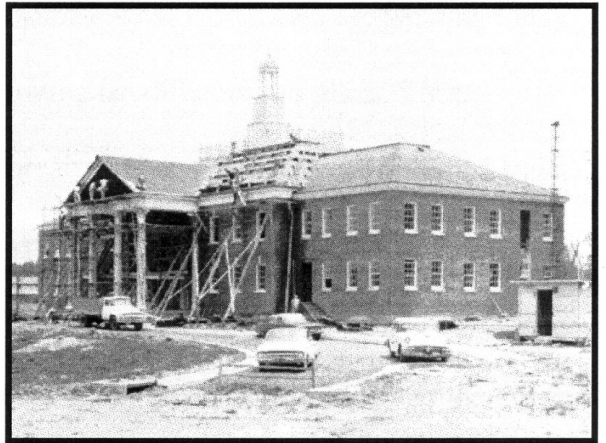
City Hall Construction, 1961
