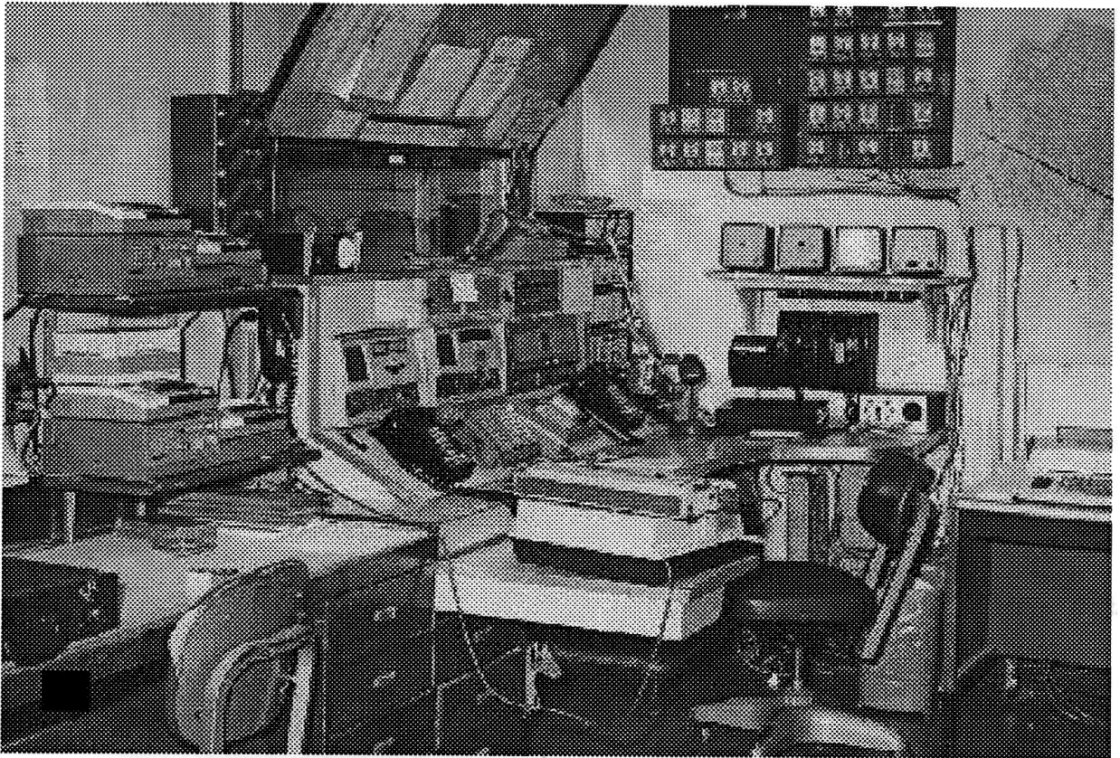
Communications Center, City Hall
